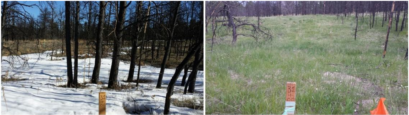
Figure 2. Before and after photos at task 2, trail corridor clearance and hazard tree removal along a future tier 1 trail route. A corridor 12 feet wide was cleared of trees and shrubs and hazard trees were removed out to a distance of 60 feet on each side. The stake indicates a distance of 3,100 feet from the start of this segment of alignment.
